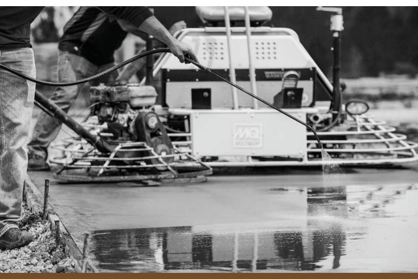
SlabArmor<sup>™</sup> Closer is a spray-on, leave-on condensifier that dustproofs and hardens in a single application with minimal clean-up.
